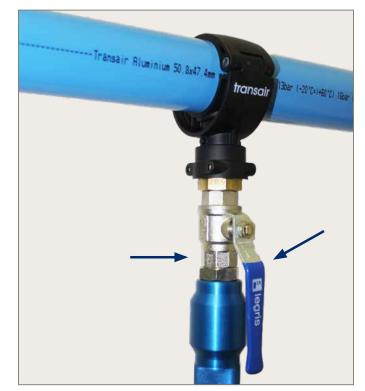
2. Thread the drilling tool onto the ball valve. Ensure the valve is open then fully drill the hole.
